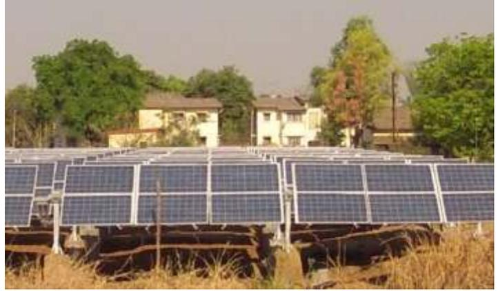
Note: The modules in this installation are oriented in portrait mode with only 4 per torque tube. This is as per design and stringing requirement of the customer.
